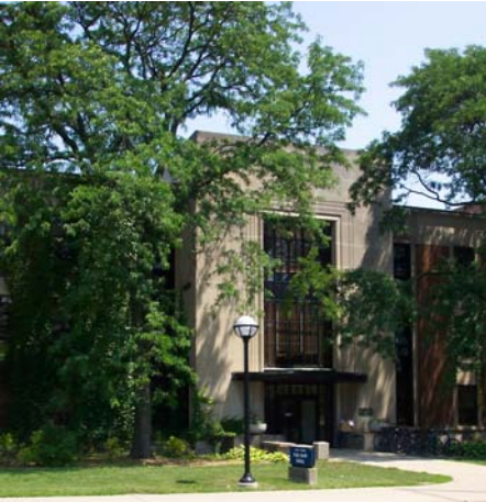
The Henry Vaughn School of Public Health Building I
